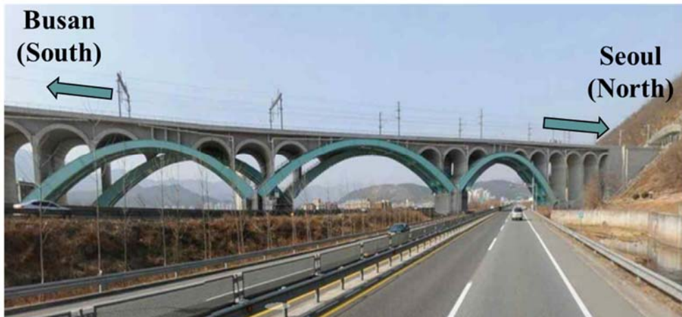
220 Figure 1. Eonyang Arch Bridge.
