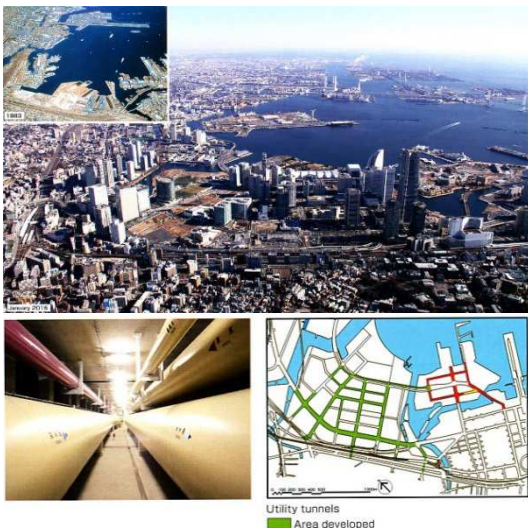
Top: Overview of Minato Mirai 21 district. Bottom: Utility Tunnel and DHC pipelines
