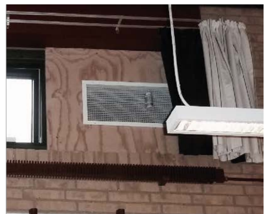
Figure 5.1.8. The system with automatic window opening and an exhaust fan – the ventilation retrofit installed in classroom S4. Window Win2 could still be opened manually by pupils and teachers.
