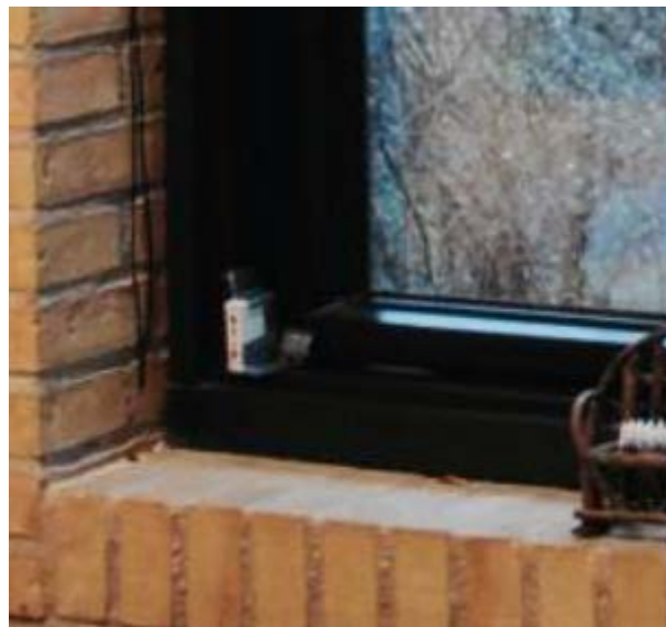
Figure 5.1.13. State logger mounted on a window frame.
