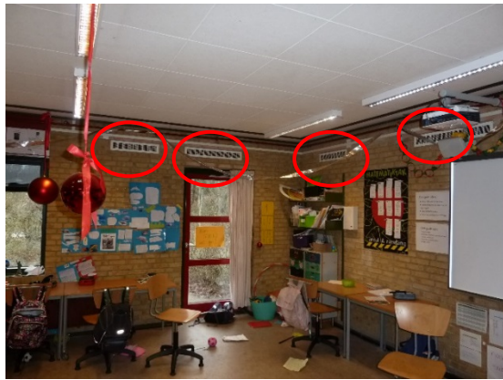
Figure 5.1.10. The system with automatic window opening and heat recovery units. Left: The units installed in the façade; Right: Red color indicates the position of all six units.
