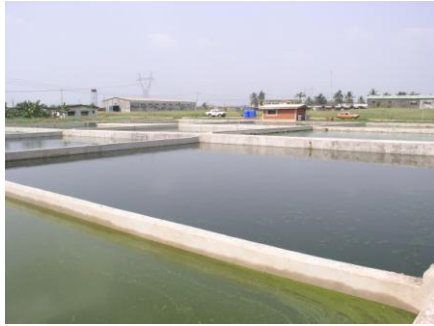
Concrete Fish Tanks are used in various sizes in Nigeria from 16 m 2 to these 380 m 2 tanks.
