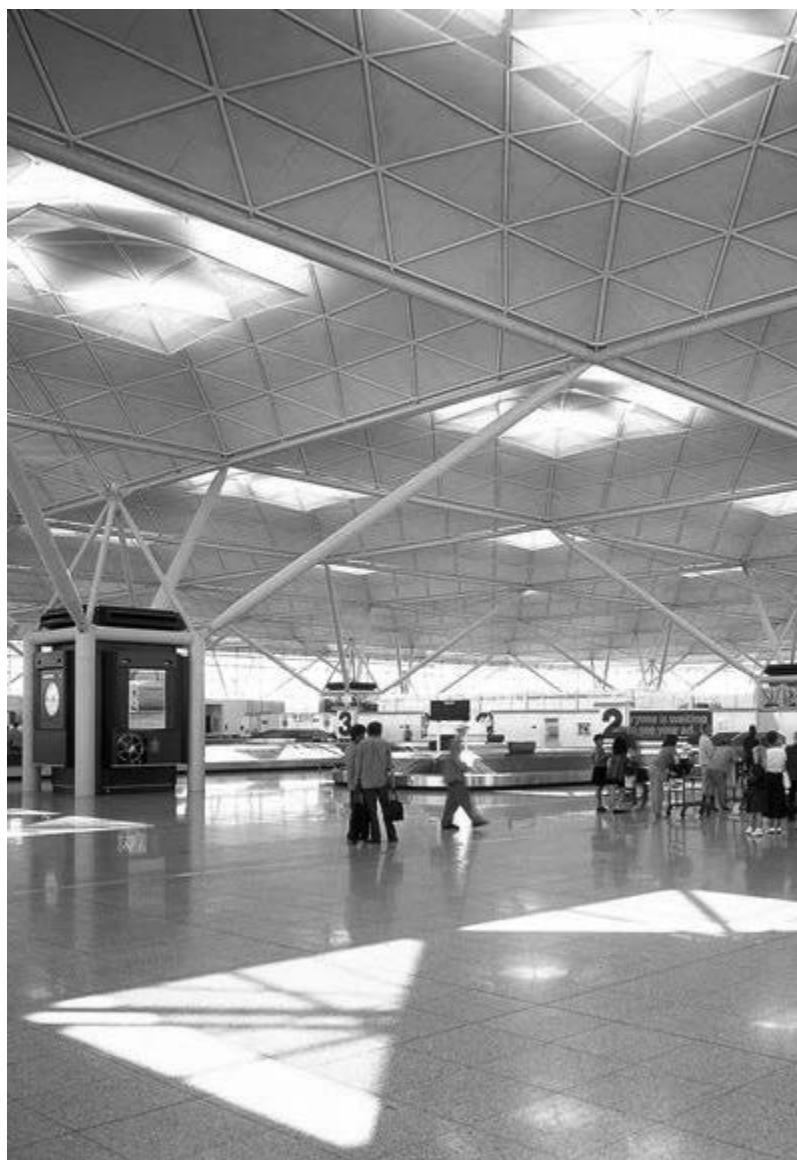
Foster + Partners _ Stansted Airport _ Stansted, UK _ 1981-91
