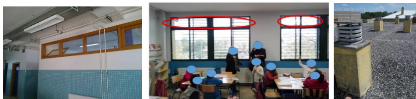
Fig. 5. Left) Cross ventilation in an Andalusian school. Right) Natural Ventilation system in an Andalusian school constructed in 1985.
