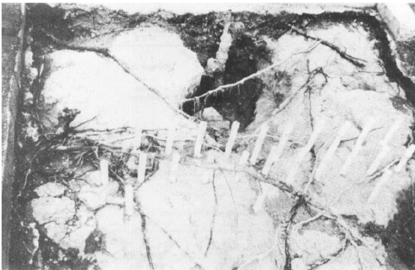
Figure 3.6. Top of caprock exposed by the removal of overburden exposed at the midslope infiltration pond site
