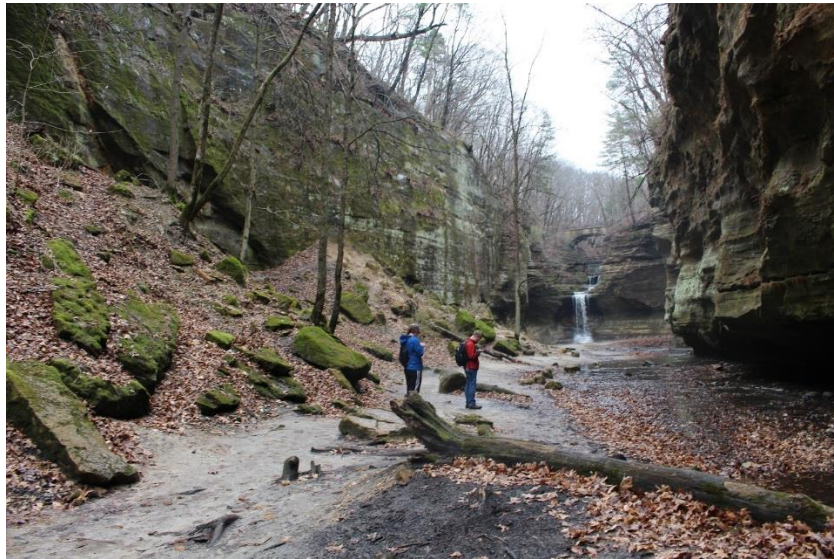
Figure 17: This photo shows one of the rockfalls that are found on the Lower Dells path. The picture also shows the 45 foot canyon walls that run parallel with the Upper Dells trail. That would be an example of a shear surface.
