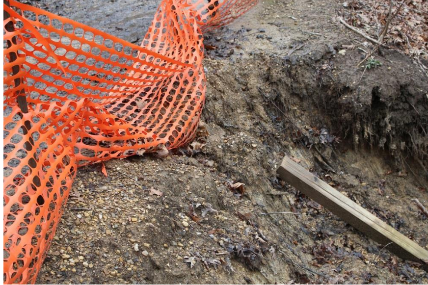
Figure 16: This photo shows a failed support. The park had to put up this orange fence to warn the public of the drop off that was created by erosion.
