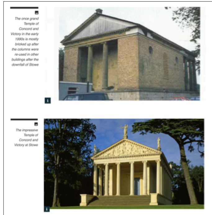
Figure 5: Renovation efforts of the Temple of Concord and Victory ("the Stowe You See Today," 2017)
