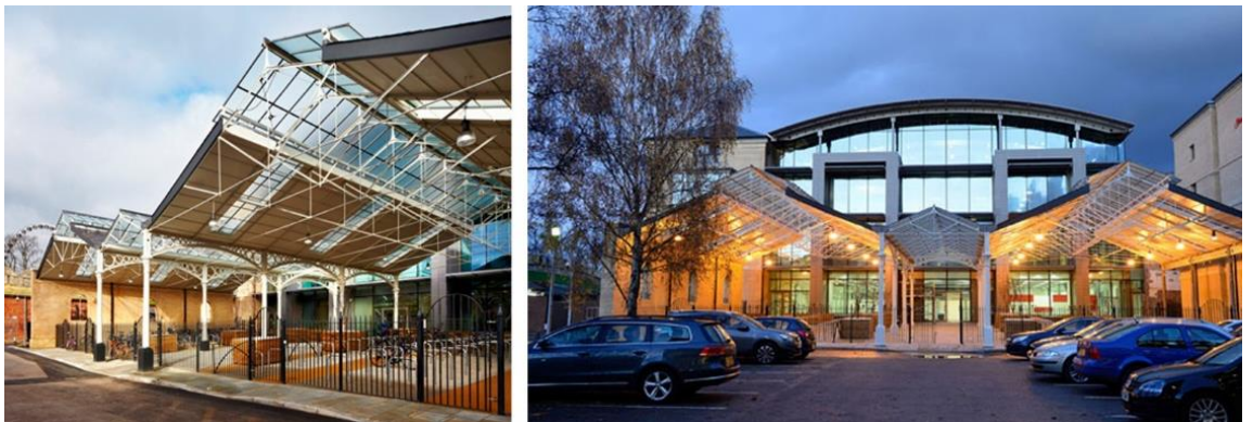
(c): The southern glazed elevation and the original train-shed relocation
