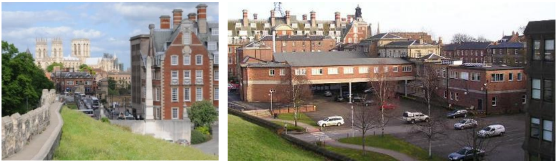
Figure 6.11: The site as it looked from the city wall before development Source: Adapted by the researcher from CYC et al. (2011)
