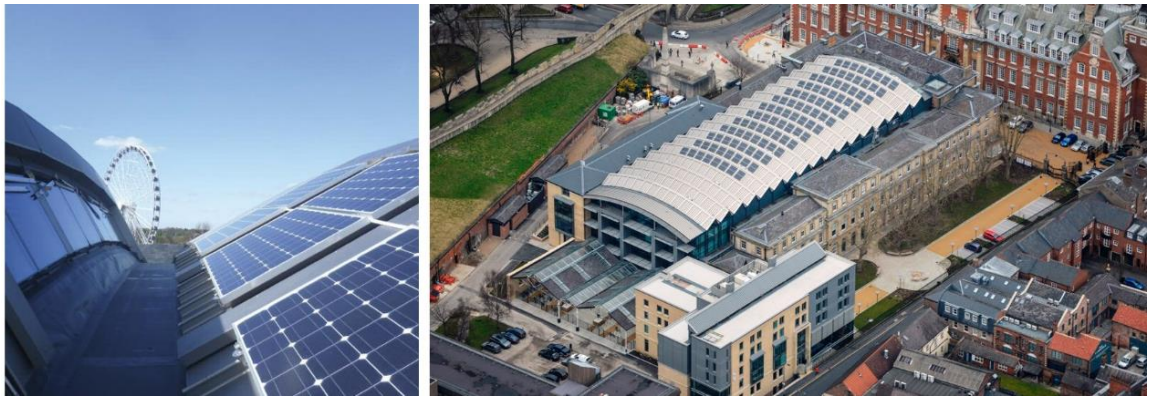
(a): The roof sky view
