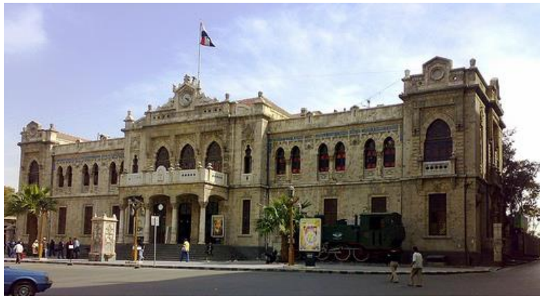
Figure 8.4: Hejaz station building Source: Asaad (2008)
