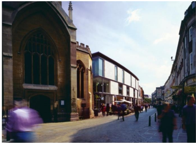
Street level elevation of Davygate Street from the west
