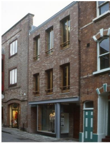
Street level elevation of Little Stonegate
