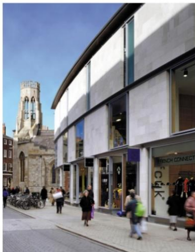
Street level elevation of Davygate Street from the east
