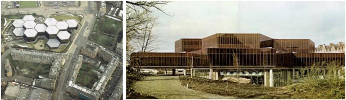
Figure 5.4: Scottish Widows' new head office at Dalkeith Road, Edinburgh, by Basil Spence. Source: www.basilspence.org.uk
