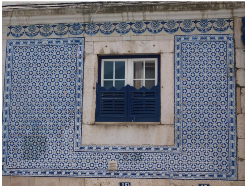
Figure 1 – Azulejos facade coating of a building in Calçada do Cardeal , Lisbon
