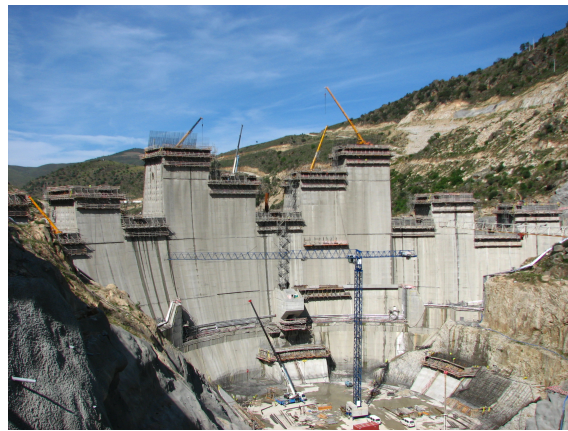
Figure 3.7: Baixo Sabor dam during construction in May 2013
