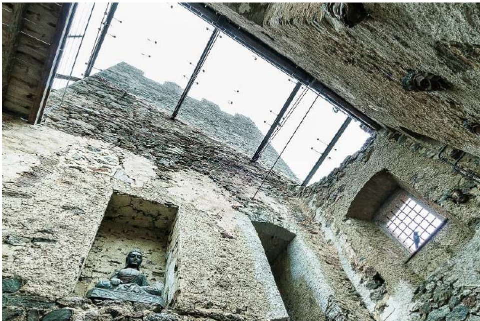
Figure 1.4: Detail of Reinhold Messner Castle's roof
