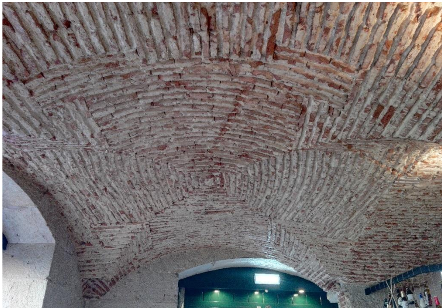
Figure 5.6 - Example of a quadripartite brick vault
