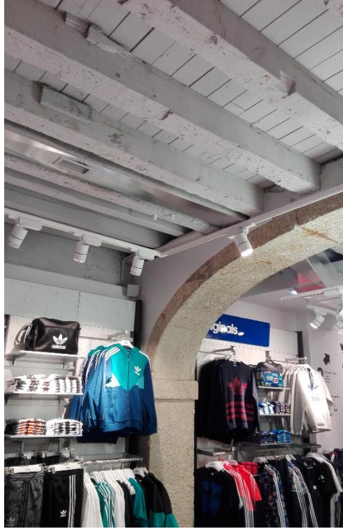
Figure 5.7 – First-floor supported in stone arches
