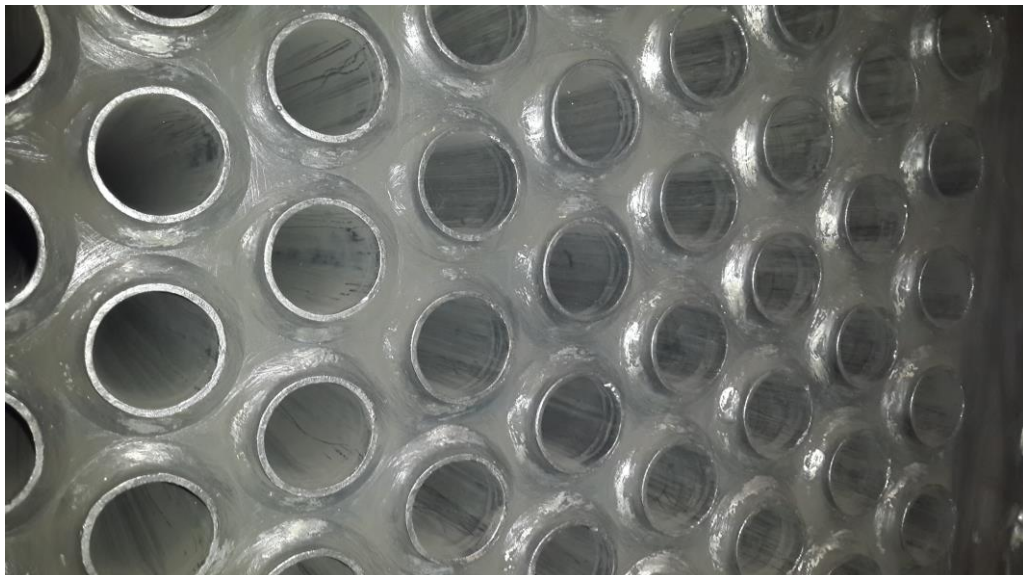
Figure 5.6 Flame tubes after maintenance work
