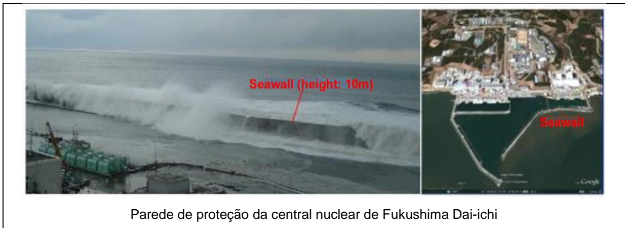
Figura 37 - Galgamento do tsunami (b) na central nuclear de Fukushima Dai -ichi (a) Fonte: Government of Japan (2011, p. III-40)
