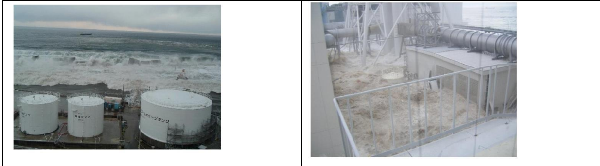
Figura 36 - Danos na central nuclear de Fukushima Dai-ichi Fonte: Government of Japan (2011, p. III-40)
