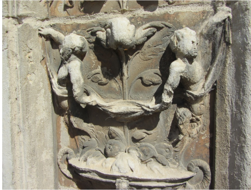
Figure 6.1: Detail of a highly decorated XVI century portal listed as Spanish National Heritage (D=5). The portal was carved in a porous dolostone and its state of decay suggests a high vulnerability (A=5). From these departing conditions, a hypothetical cleaning with nebulized water and brushing could mean: an aggressiveness of B=3; a synergy of C=1.5 for the use of water; and a synergy C=2 for the use of mechanical action, leading to a risk likelihood of 45 and an overall risk classifiable as 'Extreme'. To reduce the risk, an alternative with ammonium carbonate poultices with: A=5; B=2.5; C=1.5, would be 18.75, a substantially lower but still 'Very High' overall risk. Laser cleaning, applied below ablation and discolouration thresholds (B=1), would keep the risk at 'Medium/High'. (Image courtesy of José Delgado Rodrigues)
