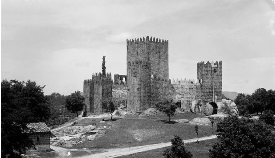
Figure 25. The Guimarães Castle after restoration works performed between 1936 and 1940. Source: SIPA
