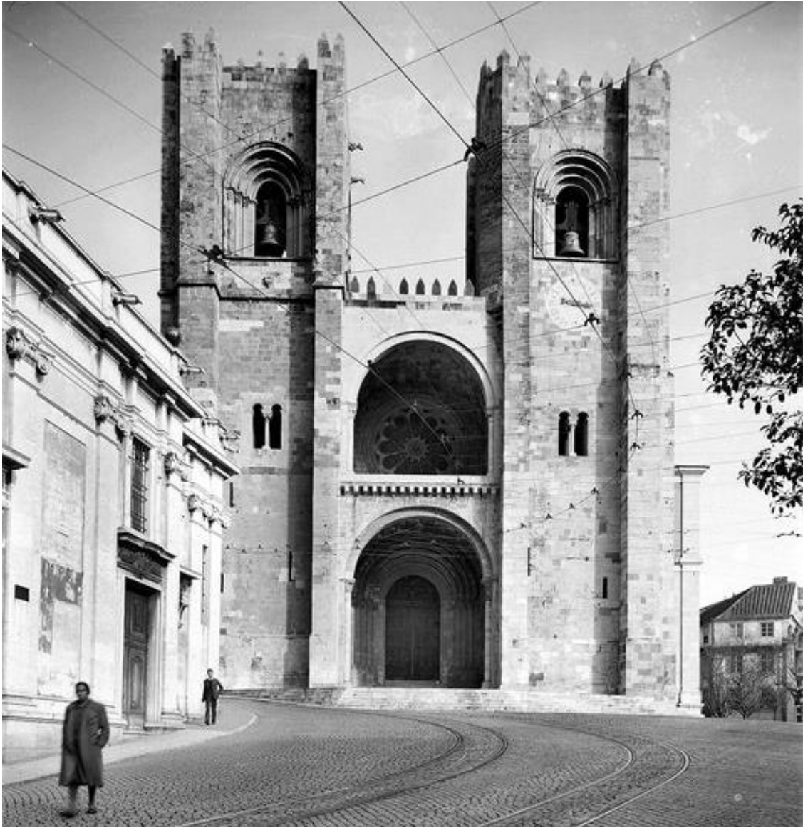
Figure 9. The same facade after the conclusion of restoration works (1939-1952). Source: SIPA
