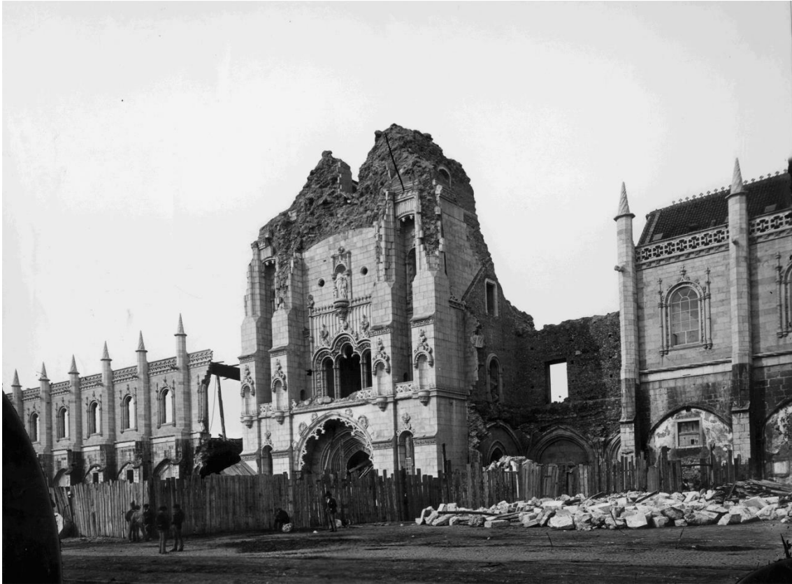
Figure 4. Collapsed tower of the central dormitory of the Jerónimos Monastery, designed by the architects Giuseppe Cinatti (1808-1879) and Achille Rambois (1810-1882). Source: Arquivo Municipal de Lisboa – Arquivo Fotográfico (PT/AMLSB/SEX/000410)
