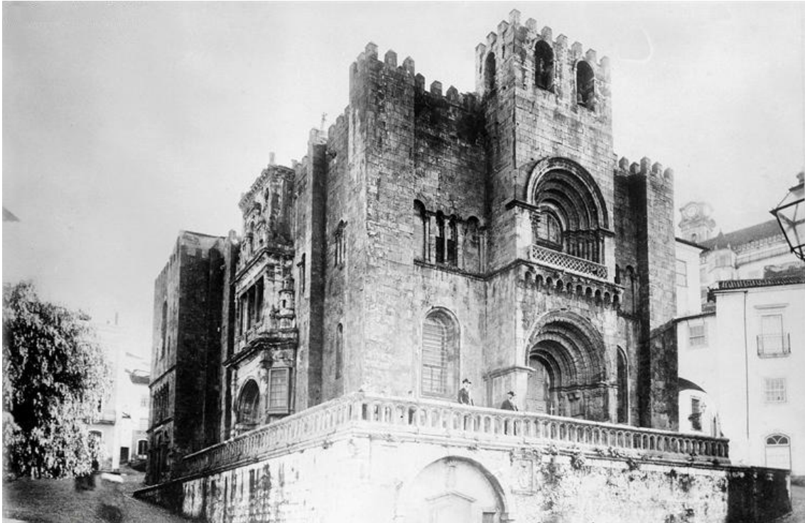
Figure 10. Western facade of the Old Cathedral of Coimbra before restoration works. Source: SIPA
