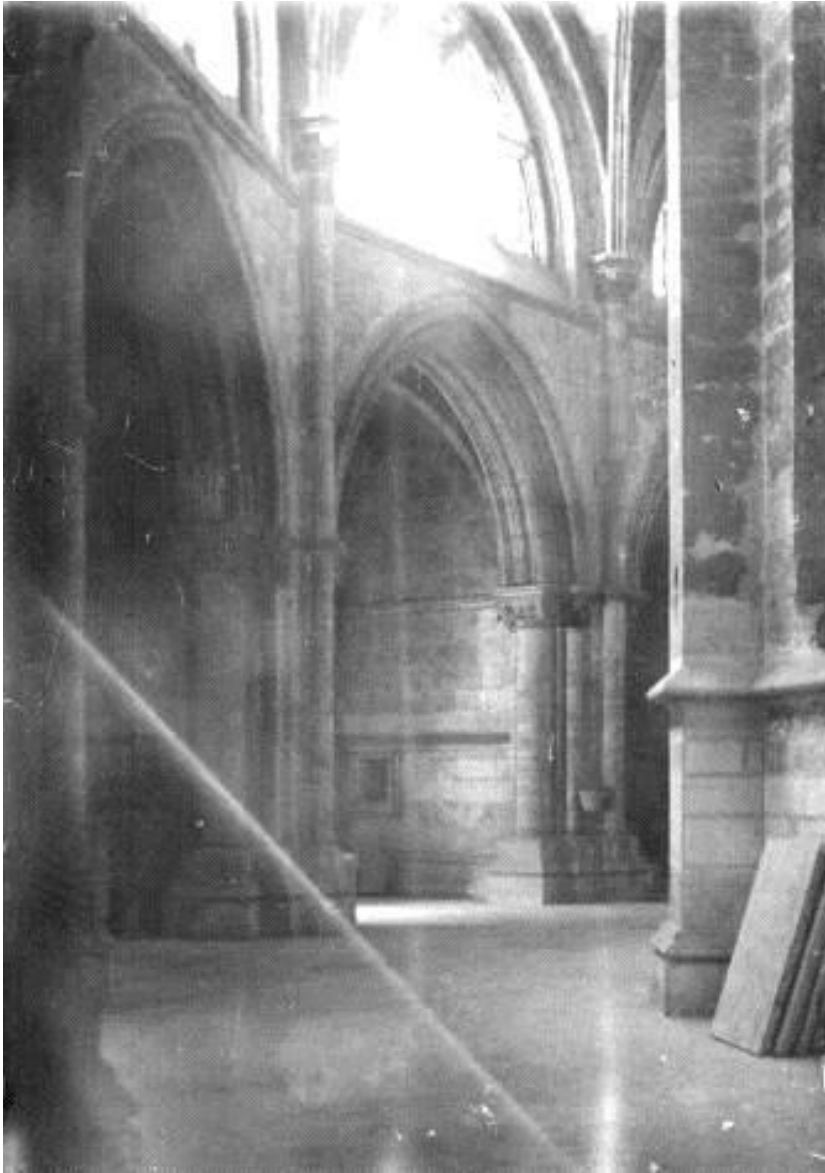
Figure 19. Ambulatory of the Lisbon Cathedral in 1925, during restoration works. Photo by Eduardo Portugal (1900-1958). Source: Arquivo Municipal de Lisboa – Arquivo Fotográfico (PT/AMLSB/POR/000458)
