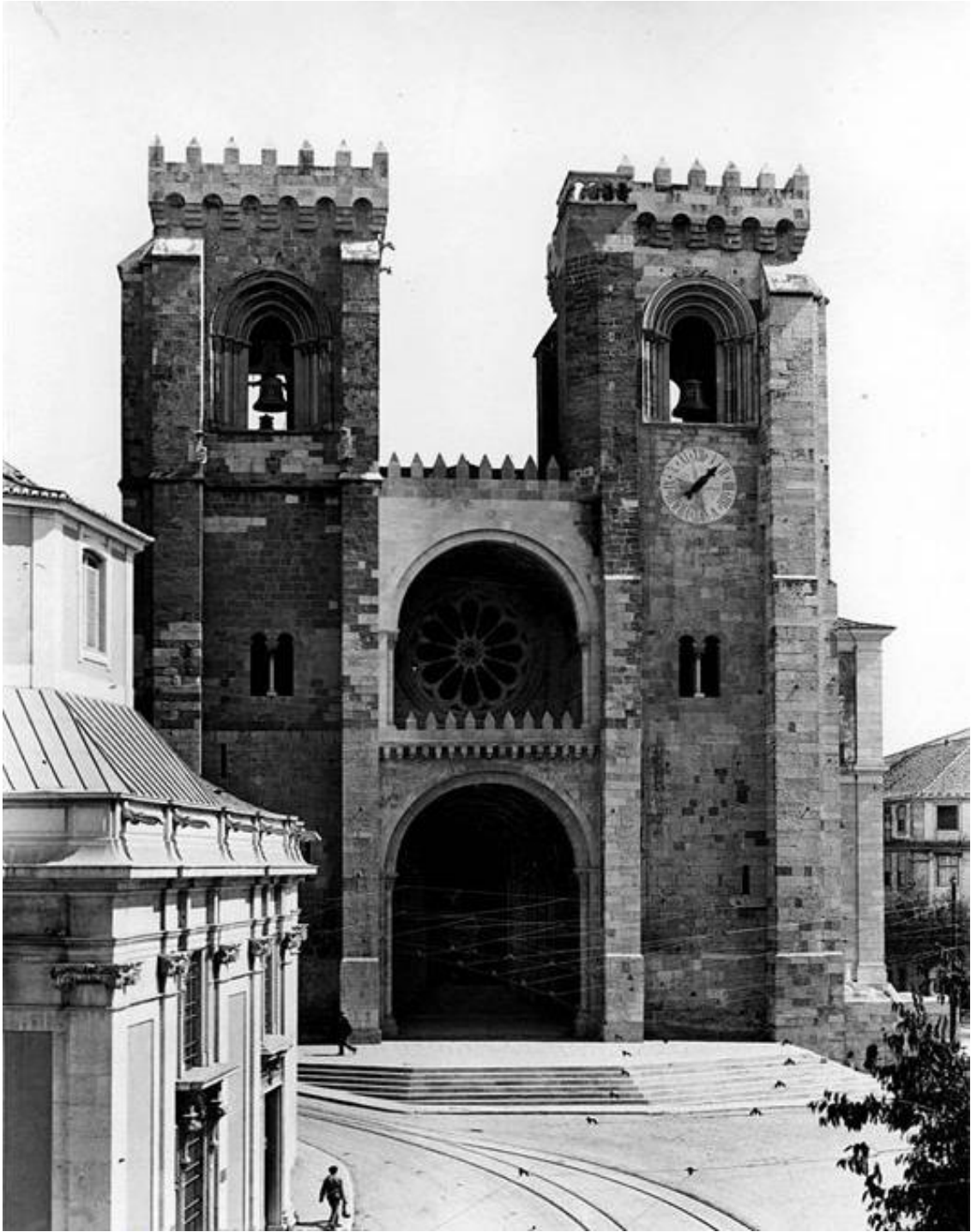
Figure 8. The western facade of the Lisbon Cathedral, after the demolition of Fuschini's pinnacles and the addition of the rose window (1929-1932). Source: SIPA
