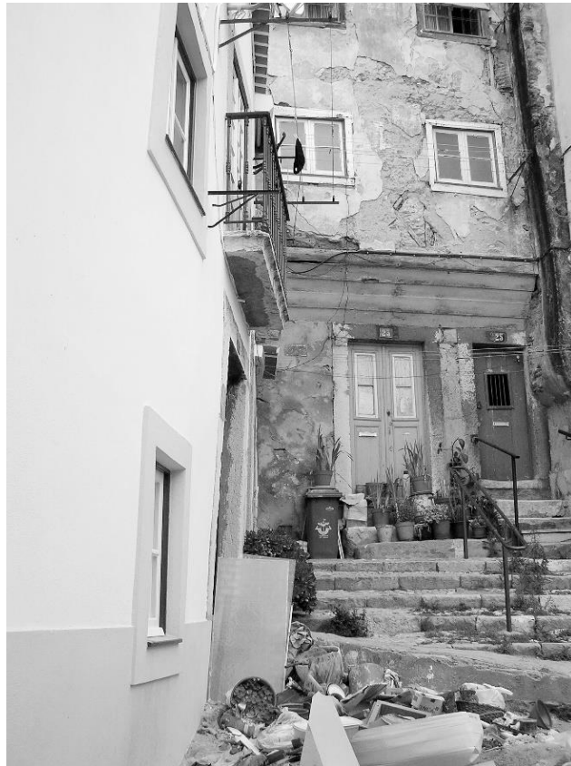
Figure 20. Decayed and rehabilitated houses, May 2012
