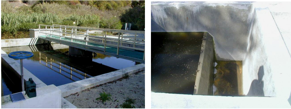
Figure 2.22 Secondary decanter
