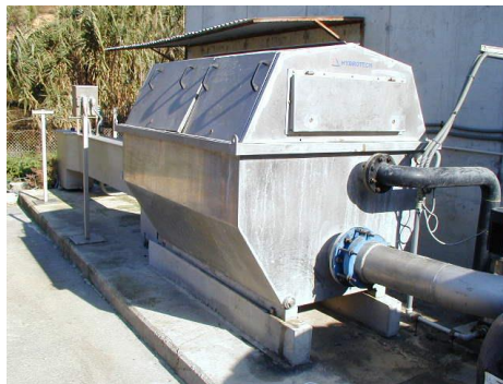
Figure 2.11 Rotary drum screen.
