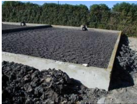
Figure 2.30 Vila Verde WWTP drying beds
