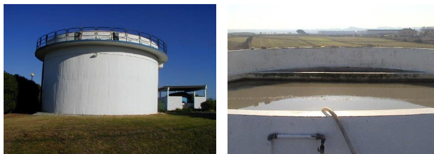
Figure 2.27 Vila Verde WWTP Imhoff tank
