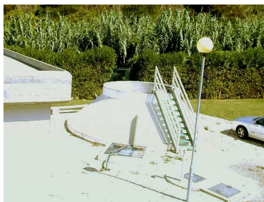
Figure 2.24 Anaerobic digester
