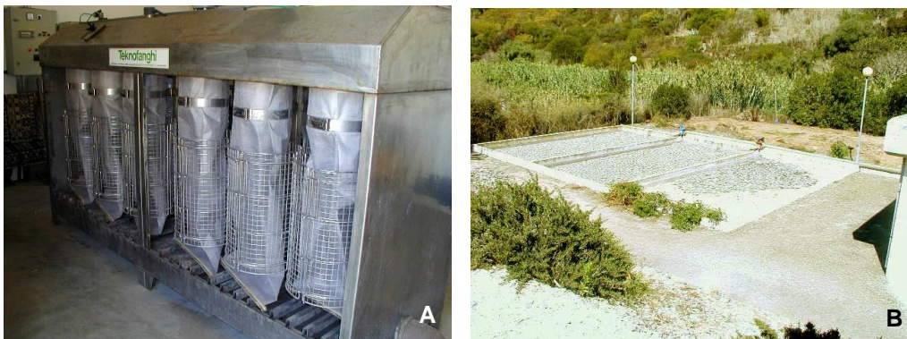
Figure 2.23 A) Filter bags; B) Drying beds
