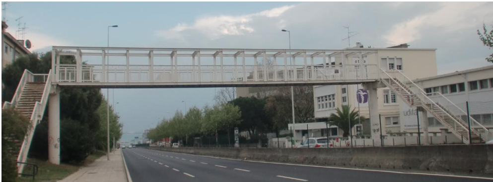
Figure 5.1: Footbridge over the Avenida Marechal Gomes da Costa, T. Krus, [15].
