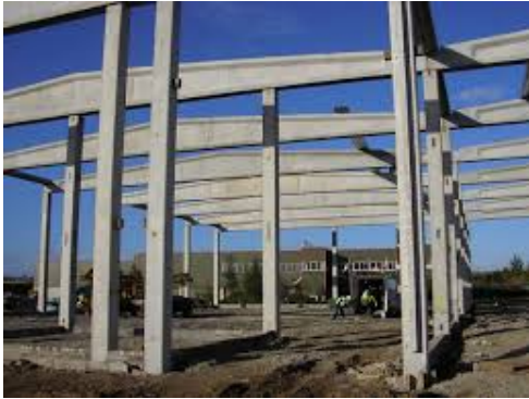
Figure 2.4.3.1 – Concrete structural frame (Shay Murtagh, 2015)
