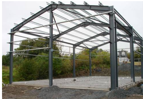
Figure 2.5.3.3 – Steel structural frame (Ecplaza, 2015)
