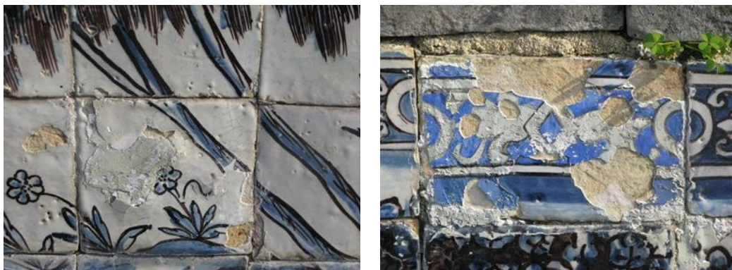
Figure 1. Lacunae infill treatments with issues of lack of compatibility, efficiency or durability. Palácio Fronteira, Lisbon, 2012. Photos by S. Pereira.
