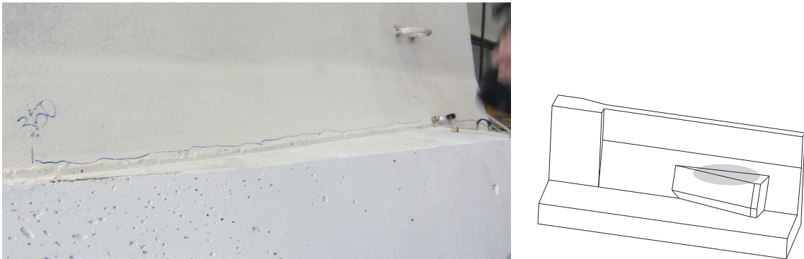
Figure 5.50: Cracking in the interface slab/blister at the fourteenth load step
