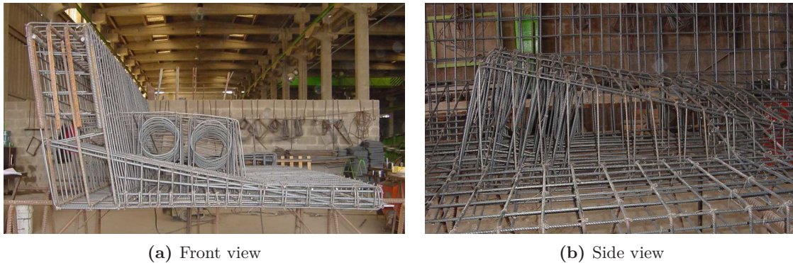
Figure 5.1: Reinforcement of the reference model anchorage blister
