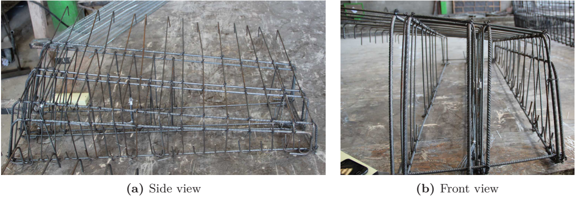
Figure 5.64: Reinforcement of the precast blister
