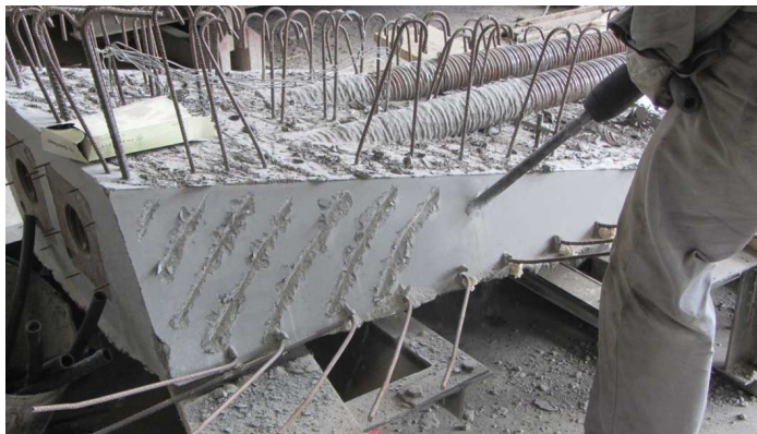
(a) Concrete surface preparation
