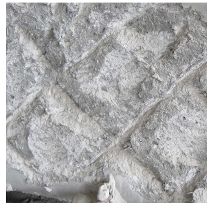
(b) Concrete surface after preparation
