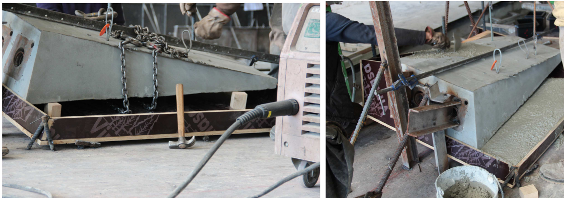
Figure 5.84: Casting of the pull-off model
