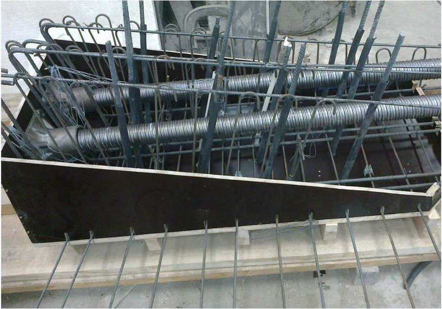
Figure 5.65: Anchorage blister ready to be cast
