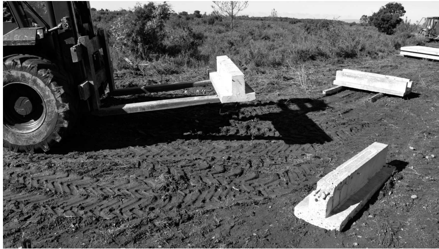
Figure 4.35: Soil beneath the supports
