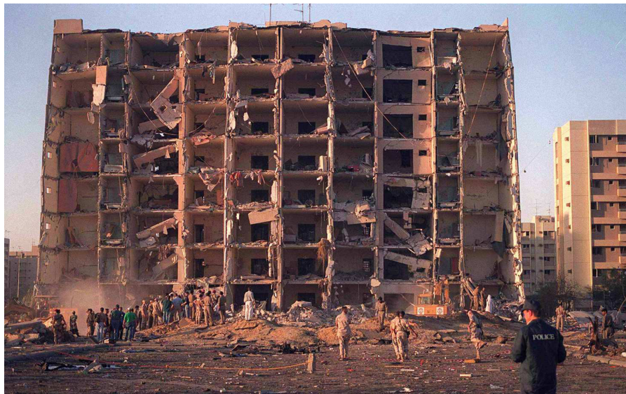
Figure 1.2: Khobar Towers damage after the bombing [42]
