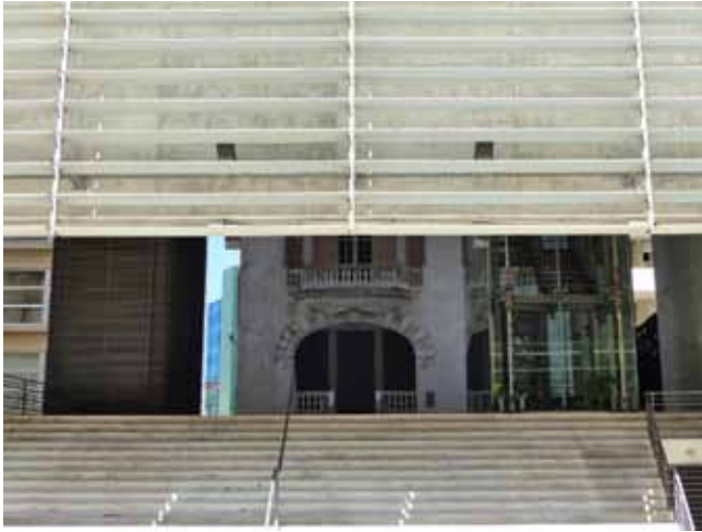
Figure 6. Headquarters of the Order of Engineers, Lisbon, rear façade (photograph provided by the author)
