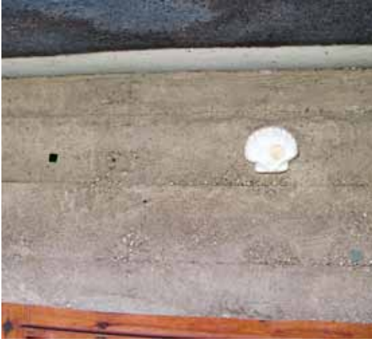
Figure 3. Detail of one of the concrete beams of the Ofir House. (Photograph by the author)
