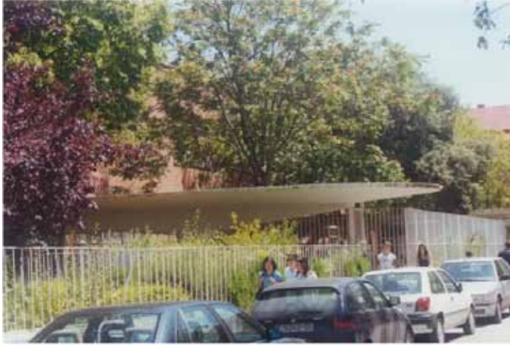
Figure 6. Projected canopy between every two classrooms of the Kindergarten of the Instituto Escuela – JAE (Madrid), 1935. Carlos Arniches. (Photograph by the author)
