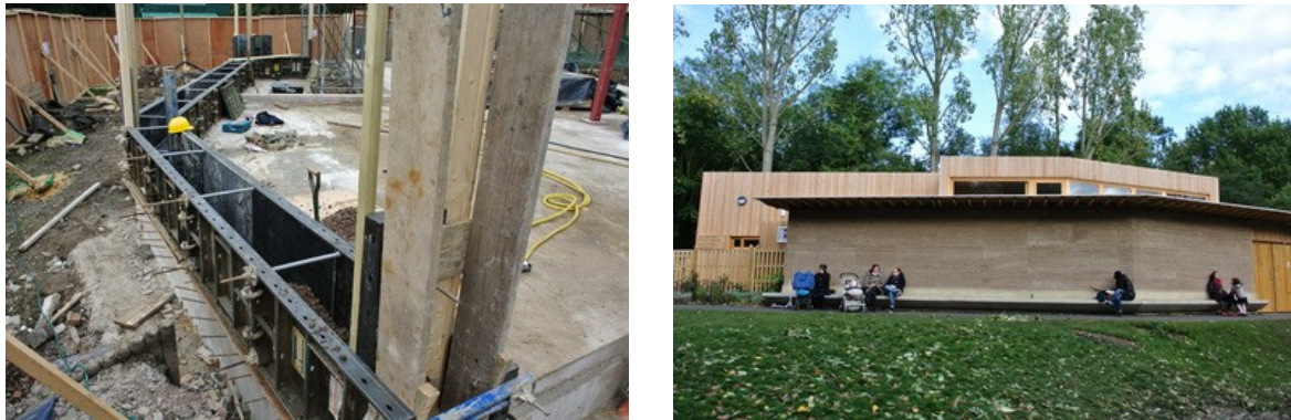
Figure 1. Earth building uses both new and old technologies, like this rammed earth in a recent project in London
