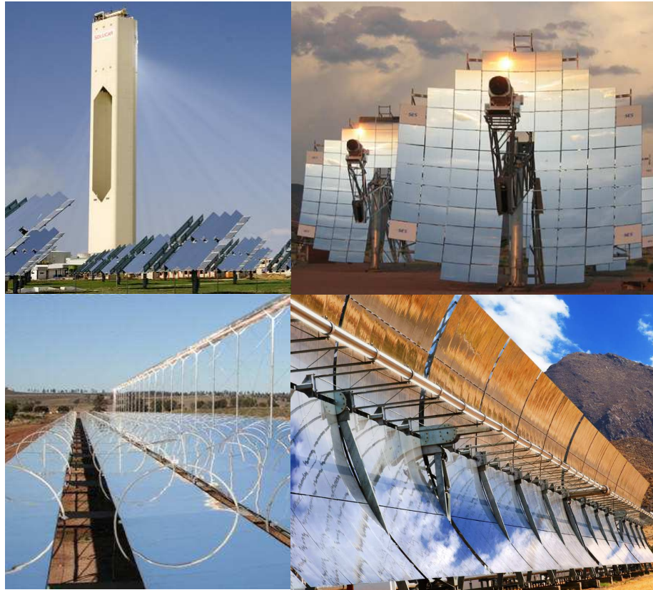
Figure 1.1: Concentrated Solar Thermal Technologies; top: Power Tower power plant PS10 in Sanlucar, Spain [2] (left) and Dish Stirling modules in Solar Two, California, USA [3] (right); bottom: Fresnel [4] (left) and Parabolic Troughs [4] (right) in Plataforma Solar de Almeria, Spain
