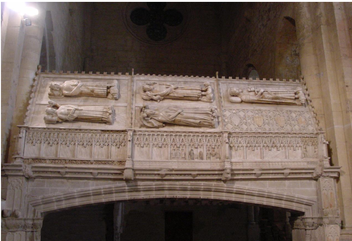
Fig. 50 – One of the burial structures of the double royal pantheon at Poblet, current view after major 19 th century restorations to open up the original arched passage underneath. The canopies had by then suffered major damages and were never rebuilt. Picture downloaded from http://ca.wikipedia.org/wiki/Reial_Monestir_de_Santa_Maria_de_Poblet .
