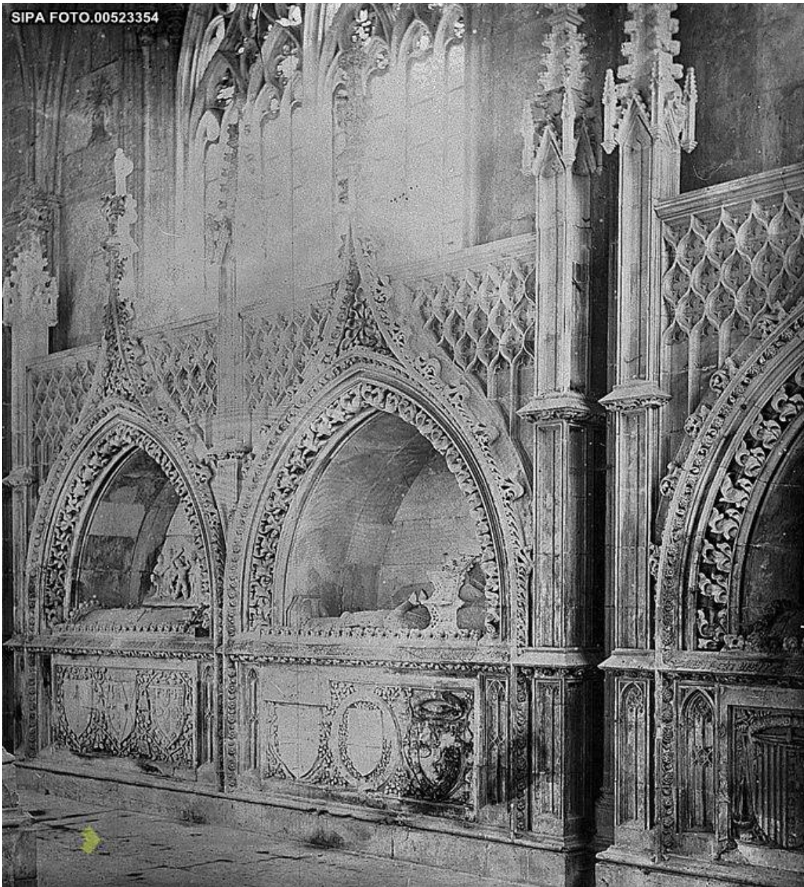
Fig. 48 – 1860 photograph of the princes' monument, with the stone relief already placed at the back of prince João's recess, before prince Henrique's front slab had been replaced © SIPA: www.monumentos.pt .
