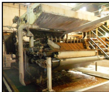
Figure 10 - View of the filter press at Portucel in Setúbal.
