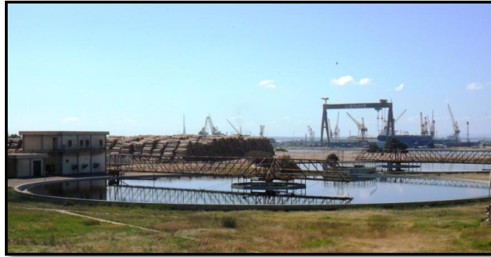
Figure 8 - View of the secondary clarifiers at Portucel in Setúbal.
