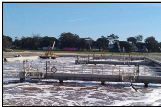
Figure 7 - View of part of the aeration tank at Portucel in Setúbal.
