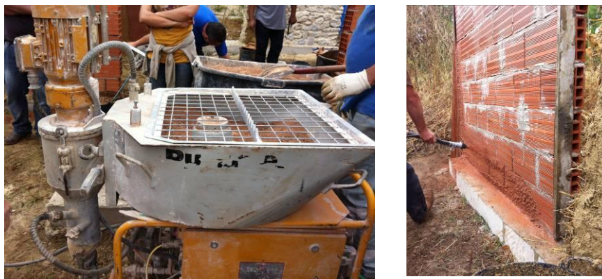
Figure 2. Mechanical mixing (left) and application (right) equipment
