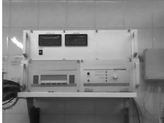
Figure C.3 - Unit controller for data acquisition by Rubotherm GmbH.
