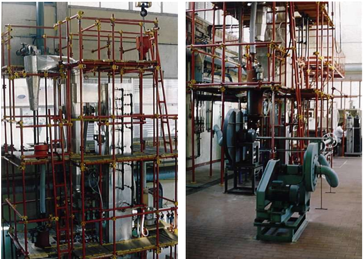
Figure 5.6 – Views of the LNEG pilot fluidised bed "New installation".
