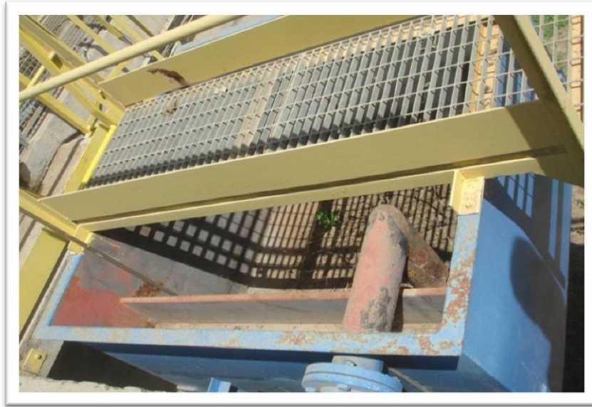
Figure 5.7 - Disused Sand Storage by source: Aqualogy Aqua Ambiente
