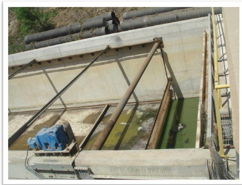
Figure 5.9 - State of preservation of Disused Primary Decanter by source: Aqualogy Aqua Ambiente
