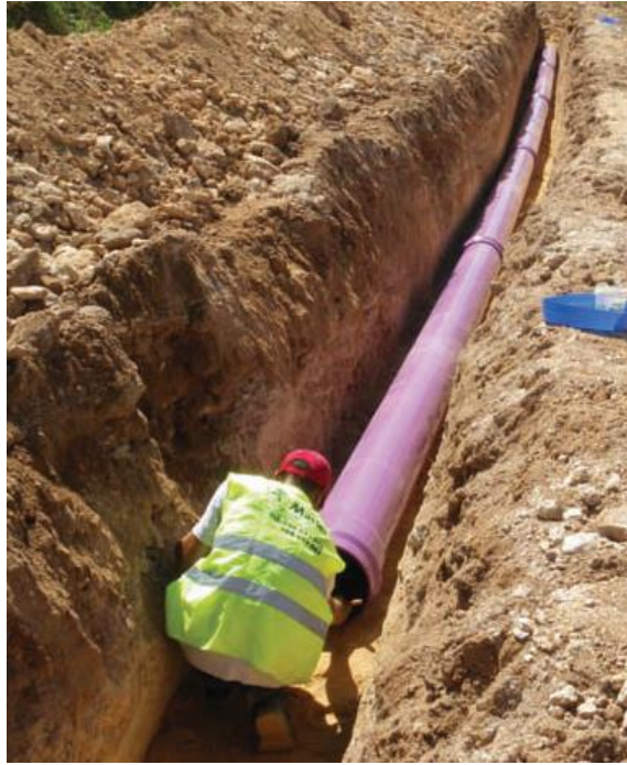
Figure 9.2 - Reclaimed water pipe in a trench; source: Aqualogy Aqua Ambiente
