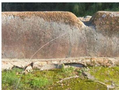
Fig. 6 and 7 – Cistern render ( frigidarium ) and detail of the opus signinum
