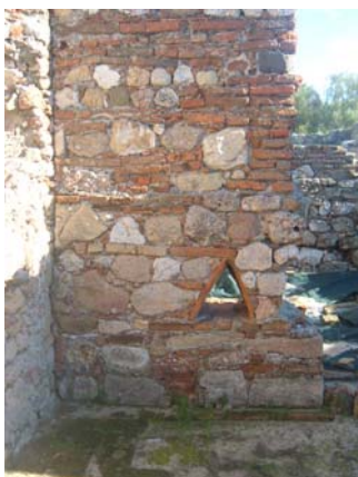
Figs. 4 and 5 - Caldarium : opus incertum and opus mixtum wall and a detail of an opus testaceum pillar
