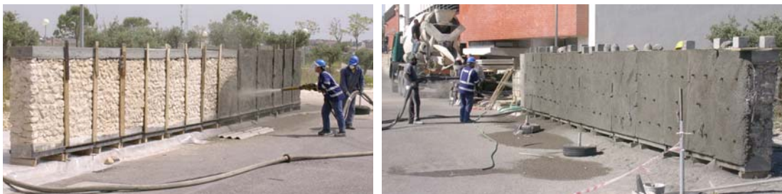
Figure 2 – Application of strengthening solution II, with mechanical methods
