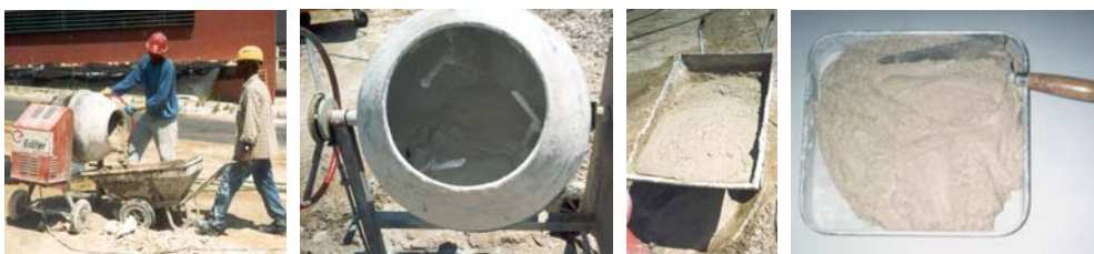
Figure 4 – Lime mortar production using a mechanical mixer
