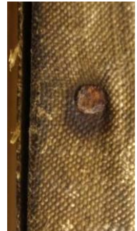
Figure 3: The tacks were in poor condition (rusted). The tacking margins of the lining fabric were deteriorated (brittle), extremely dirty, with poor attachment, in part due to the condition of the tacks.
