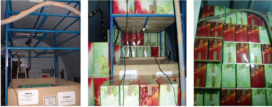
Figure 7.21: water shield (L > R) before, during, and after construction.
