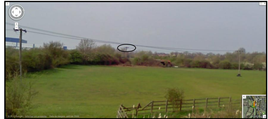
Appendix Figure IV.6 - 150 ACSR OHL in the distance.
