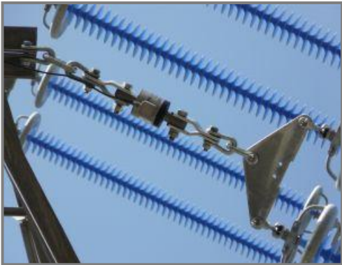
Figure 5.1 - Tension measurement [www.nexans.de].
