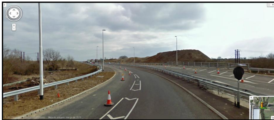
Appendix Figure IV.3 - 150 ACSR OHL crossing the first highway through an underground section with pole 17 on the right and pole 16 on the left.
