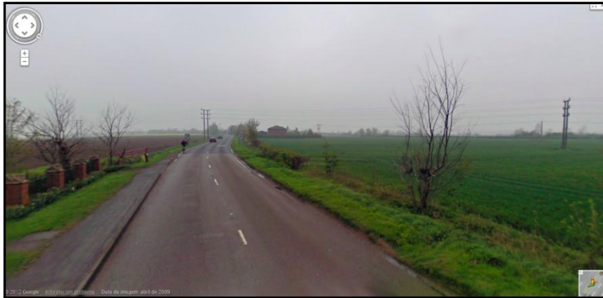
Appendix Figure III.1 - 200 ACSR OHL with pole 5 on the right and 6 on the left.
