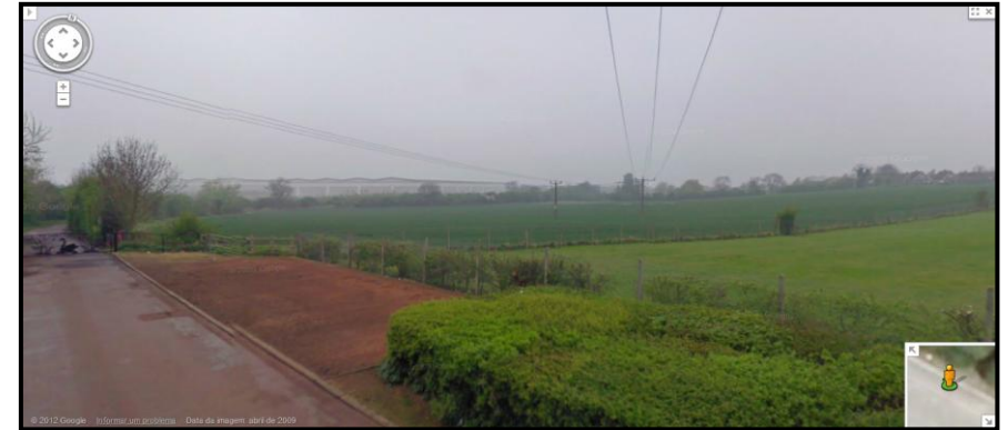
Appendix Figure IV.2 - 150 ACSR OHL crossing a field with pole number 24 in sight. No visual obstruction of notice.
