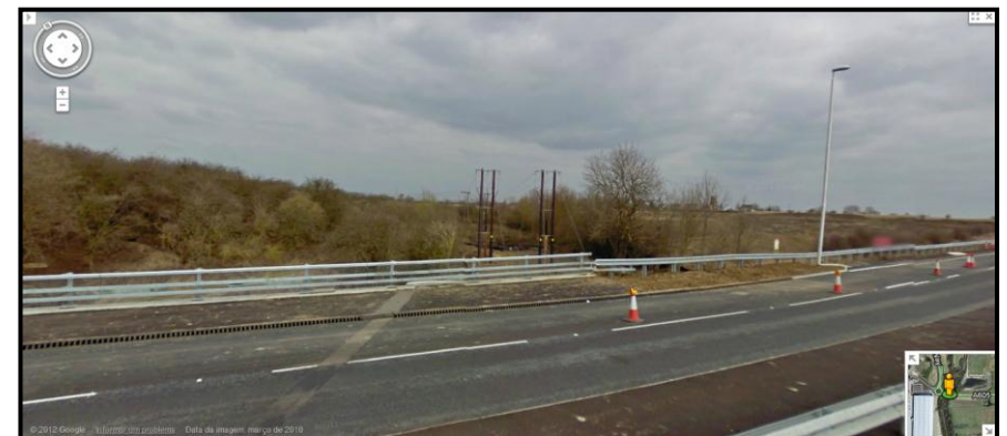
Appendix Figure IV.4 - 200 ACSR OHL after first underground section with pole 16 on sight.
