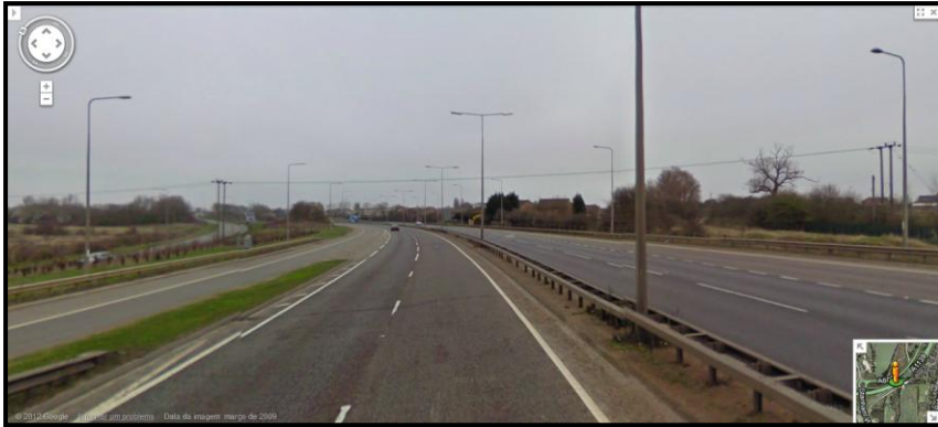
Appendix Figure IV.5 - 200 ACSR OHL crossing the second highway with pole 11 on the right and pole 10 on the left.
