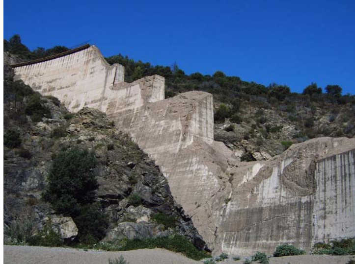
Fig. 1.1 – Malpasset dam, failed in 1959 in France
