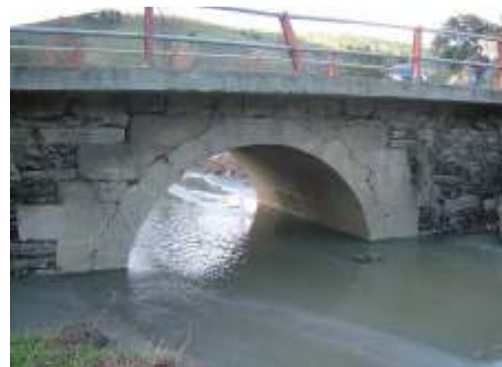
Figure 22. View from the bridge from upstream (Section 29).
