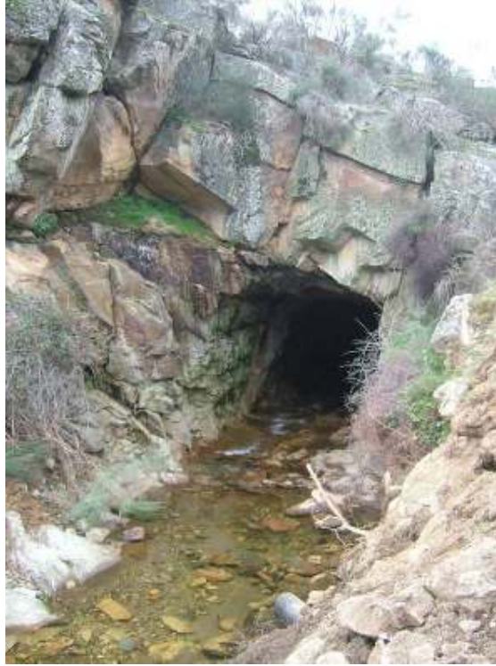
Figure 9. Upstream section of the spillway.
