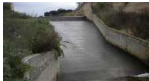
Figure 4. Spillway of Herdade da Misericórdia dam of the rehabilitation (2011).
