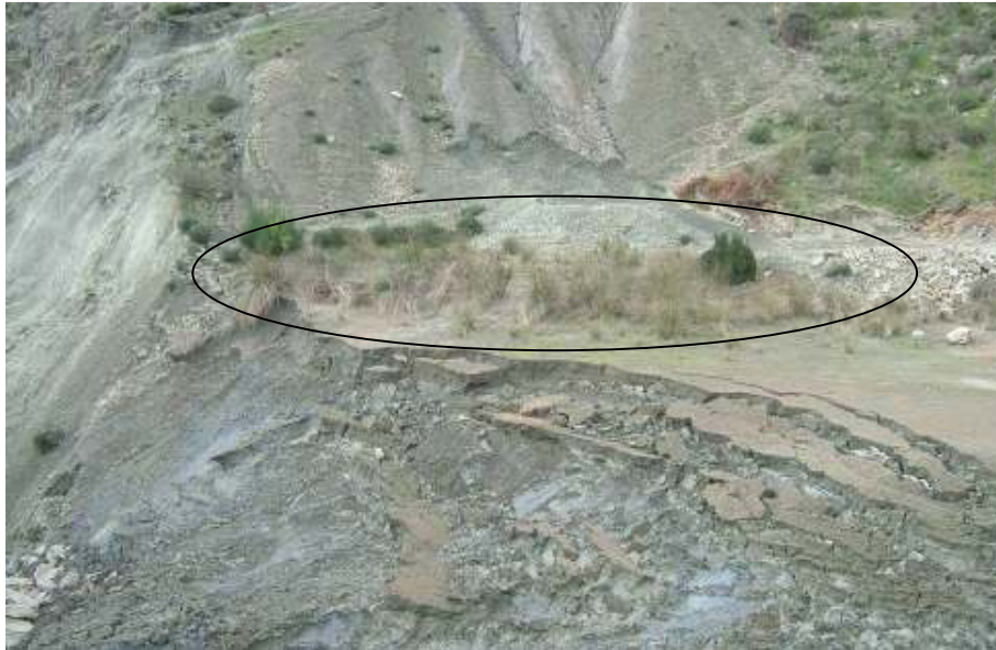
Figure 12. The remains of the dam slope and the wedge mud (at elevation 501 m asl). Dry bushes due to submersion in the winter season indicated with the black line.
