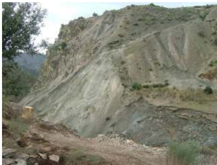
Figure 18. Dam breach, view from upstream. The wedge of mud is visible.
