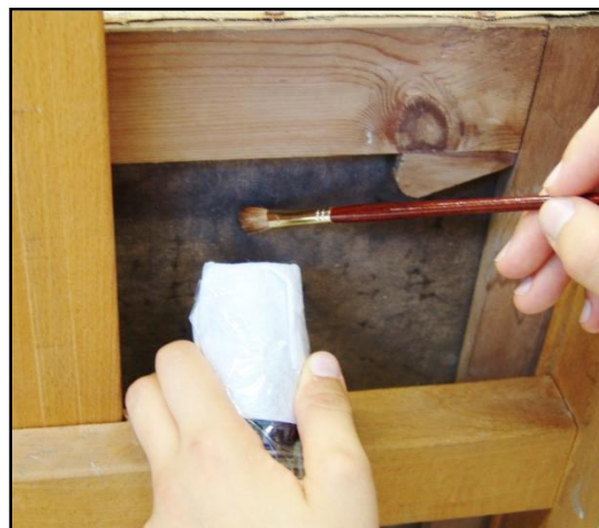
Fig. V.3. Normal light photographic detail of mechanical cleaning
