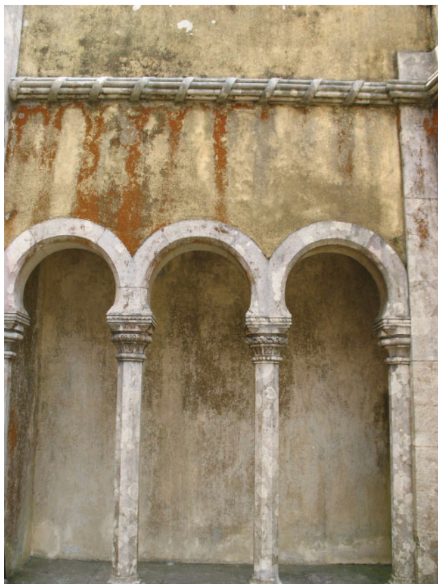
Fig. 1. Wall of the Palácio Nacional da Pena, Sintra (Portugal), showing extended colonization by Trentepohlia sp.
