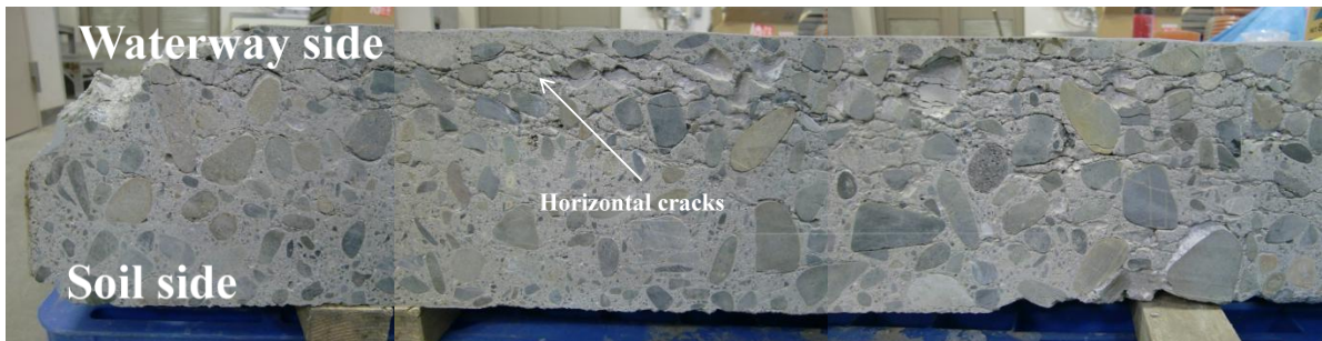
Fig. 3 Overview of local crack distribution of core sampling wall.
