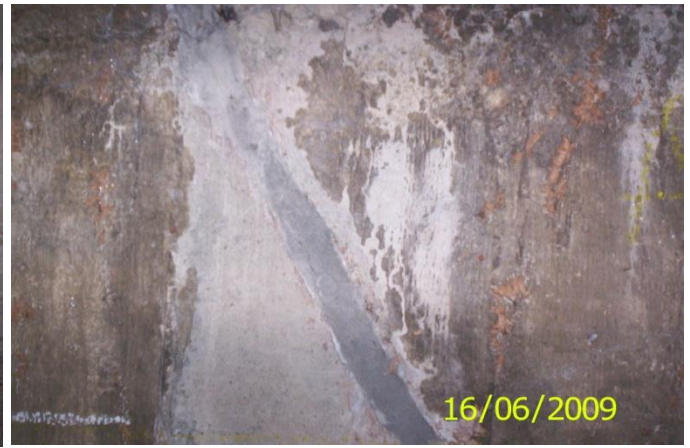
Figure 6 Minor repair on the structure
