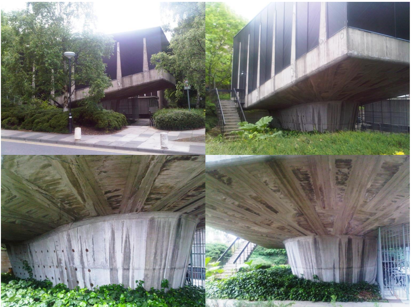
Figure 1 Engineering Lecture Theatre
