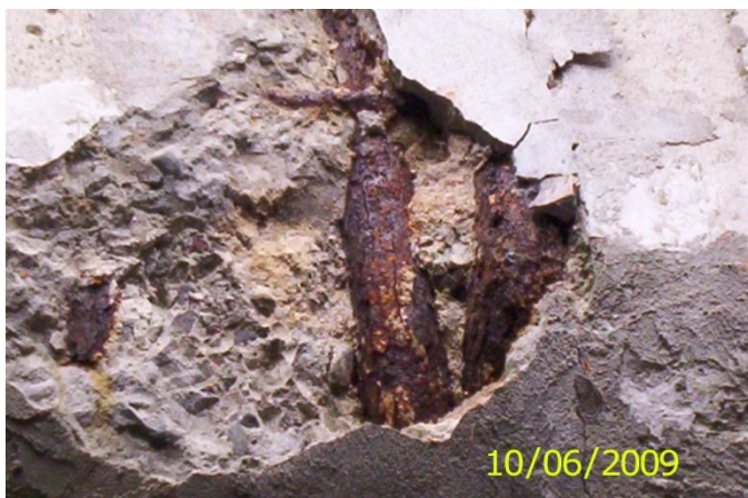
Figure 3 Exposed reinforcement
