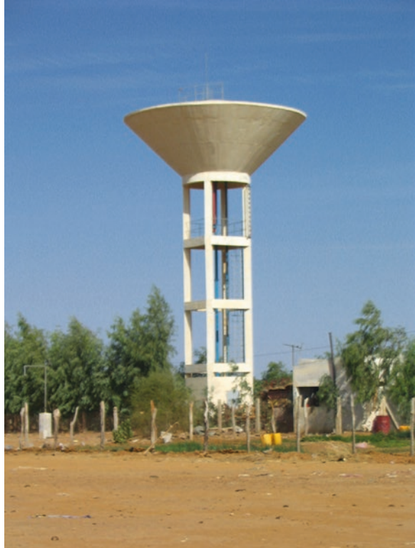
Fig. 6.9 The forage (water borehole and storage tank)
