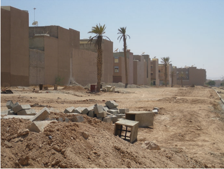
Fig. 6.4 A new housing development under construction on the outskirts of Tiznit
