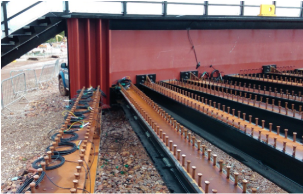
Figure 1. Installation of fibre optic sensors on bridge
