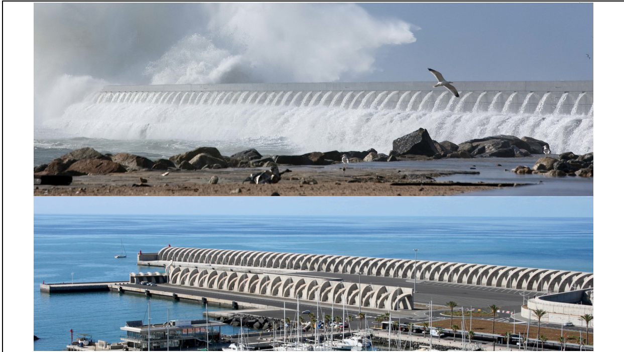
Figure 11: Landscape comparison: Natural parabolic waterfalls in “Molhe Norte da Barra do Douro” Porto (up) vs. elliptic crown wall in Tazacorte (down)
