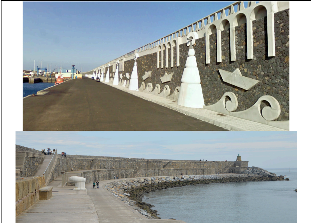
Figure 13: Aesthetics in the inner crown wall with other materials. Punta Restinga (up) and Zumaia (down)
