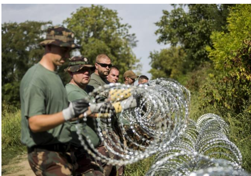
Figure 6. construction of Temporary Border Fence started on the Hungarian border [17]
